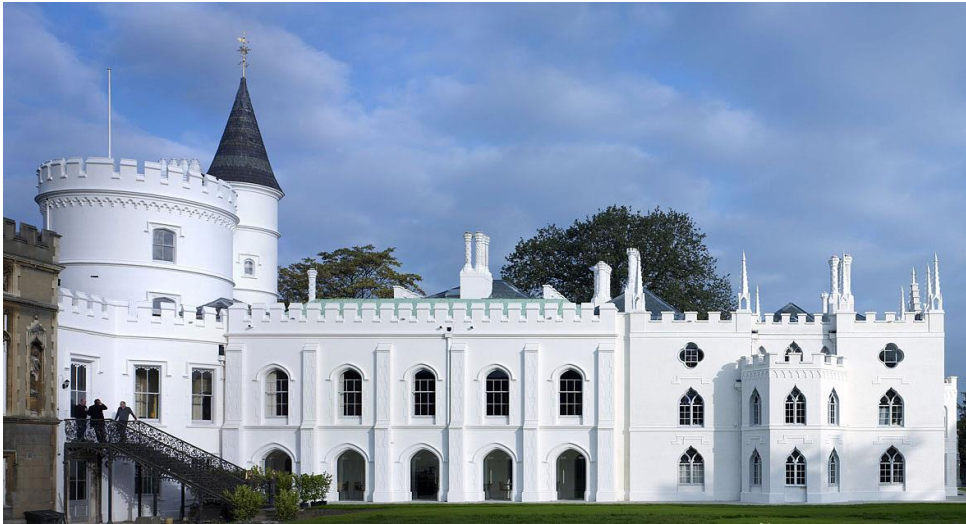
Strawberry Hill House after restoration in October 2010
